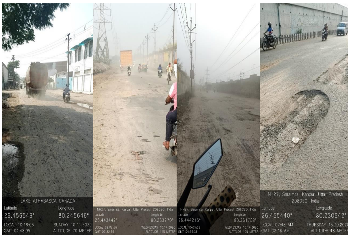
Figure 3.100: Broken roads causing higher road dust emissions
